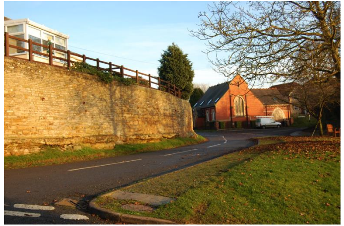
Substantial stone wall at No 13 High Street
